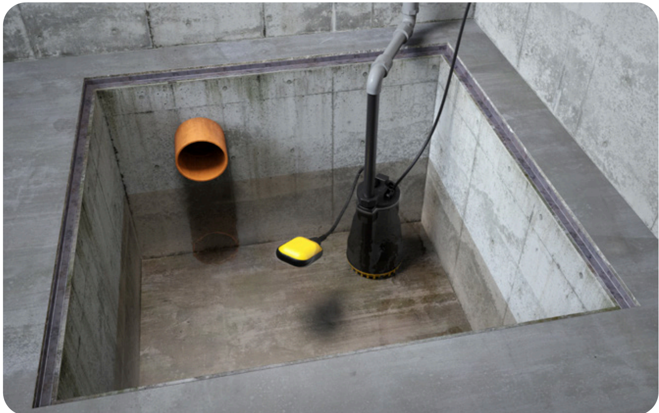
Fig.: Submersible pump ZM A with float switch in pit
